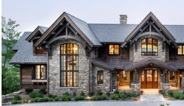
Example of home where metal roof is ancillary to main roof material
