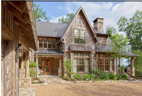
Example of home with articulated metal roof
